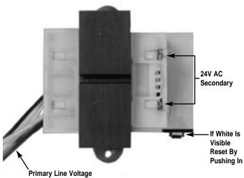
6. If 24V AC is present the electronic control board may be defective.
